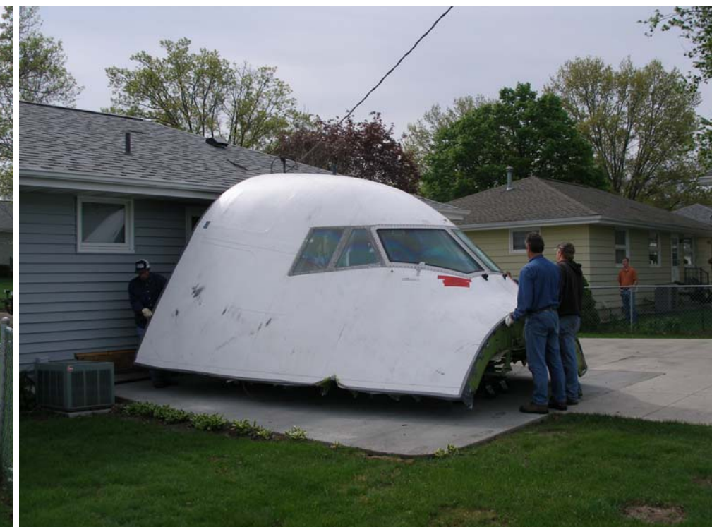
When the cockpit was put into place, a car jack was used to lift the corners to remove the dollies and the cockpit rested on wood blocks.
