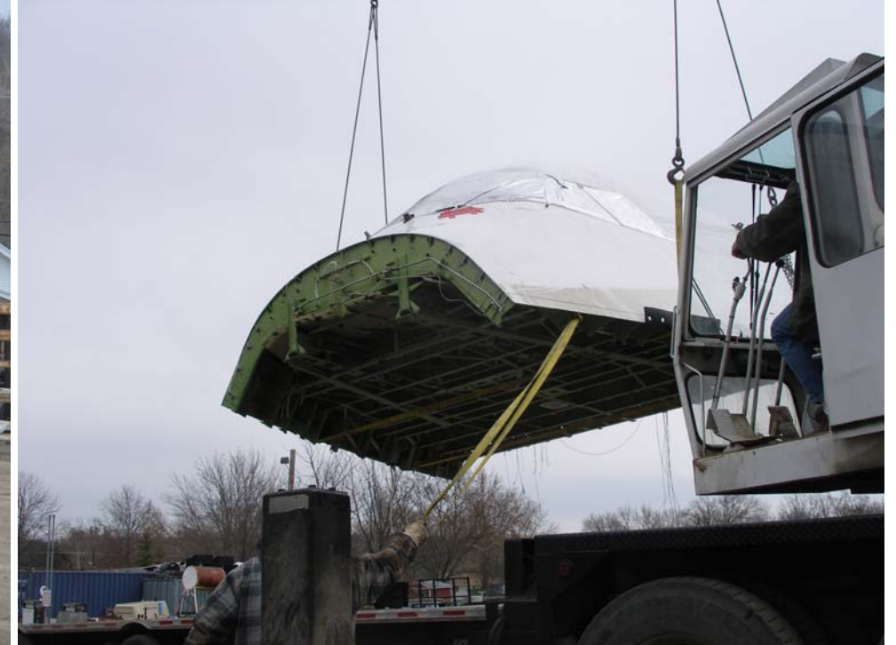
Crane removal from flatbed truck
